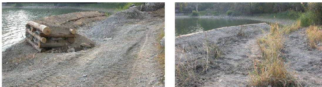
Figure 3: Riparian restoring action with living palisade and laying of reed bed (source: Aimone, 2014)
