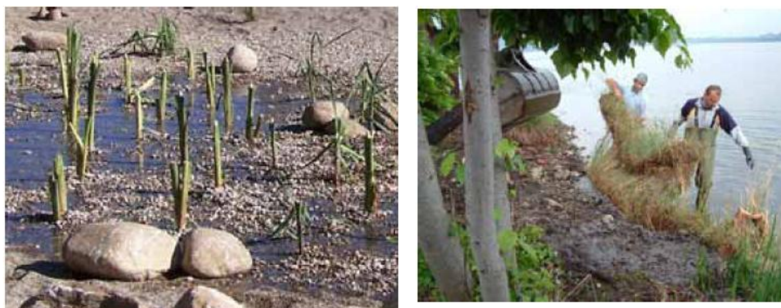
Figure 4: Reed installation with clods (on the left) and installation of reed coconut rollers (on the right) (source: AA.VV. 2011 – Quaderni della ricerca n. 125 - Regione Lombardia)
